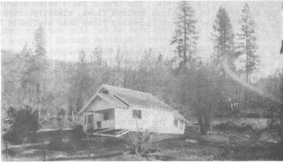
Figure 10. The 1955 flood destroyed many homes and tourist cabins. This one was moved from its foundation and severely damaged.
