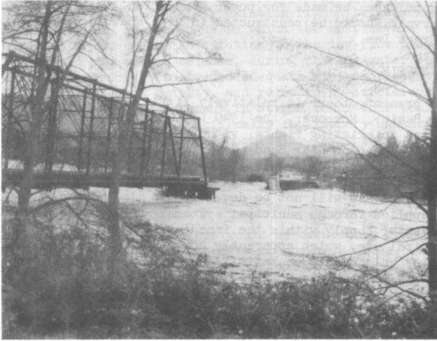
Figure 8. Railroad bridge at Grants Pass, destroyed by 1955 flood, shortly after peak stage.
